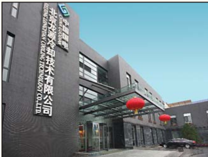
Beijing Longyuan Cooling Technology Company, Beijing, China
