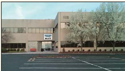
EVAPCO-BLCT Dry Cooling, Inc. Divisional Headquarters, Bridgewater, NJ
