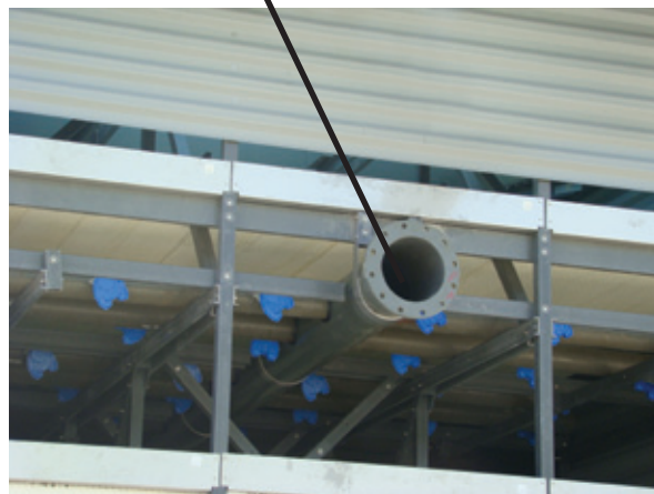
Fire-retardant water distribution system header and branch arms
