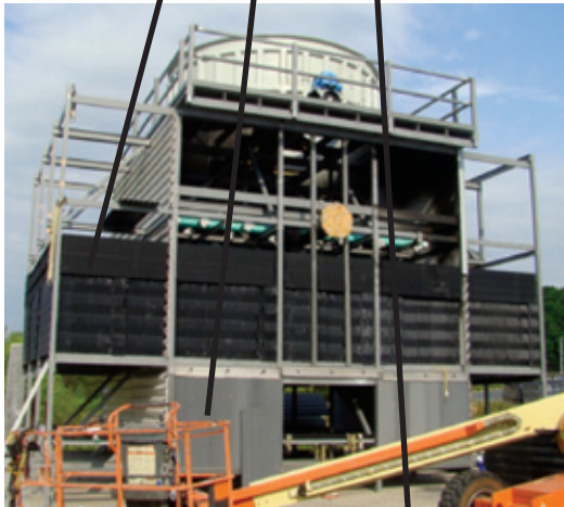
Series ES test cell under construction with standard PVC fill, eliminators, and WST inlet louver panels
