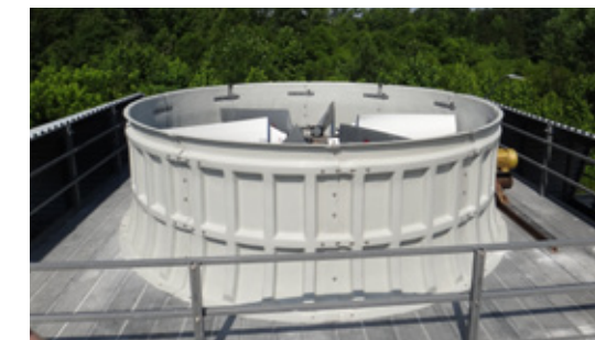
Series ESX test cell under construction with FR fan cylinder.
