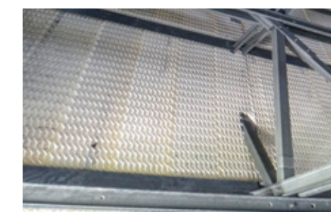
Series ESX FM test cell with Franklin™ eliminators
