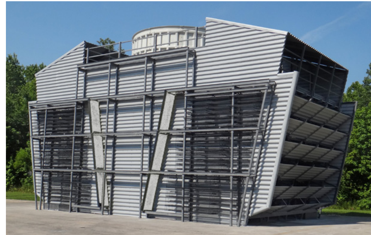
Full scale Series ESX crossflow FM test cell.
