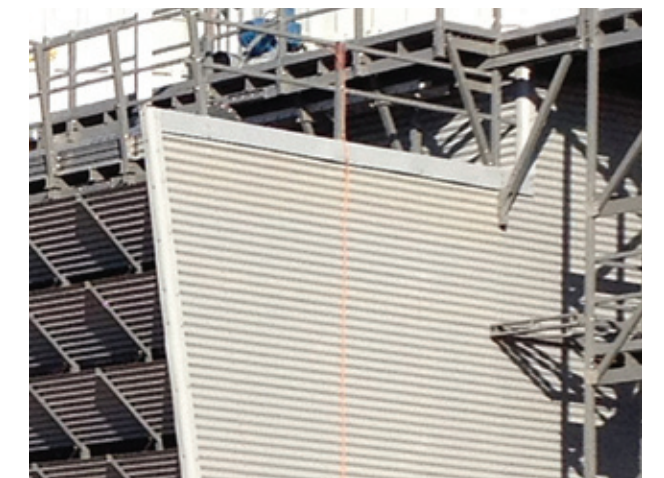
Series ESX SafeWall™ custom fire retardant fiberglass casing and partitions..
