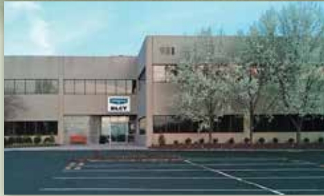
EVAPCO-Dry Cooling | Bridgewater, New Jersey
