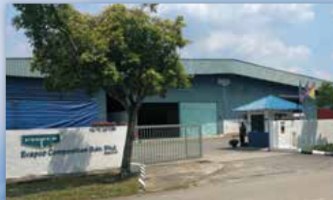
EVAPCO Composites Sdn. Bhd Selangor, Malaysia
