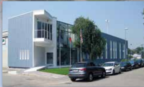
EVAPCO Europe, S.r.l. | Milano, Italy
