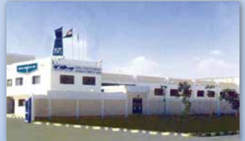
Evap Egypt Engineering Industries Co. | Cairo, Egypt
