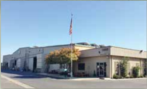
EVAPCO West | Madera, California
