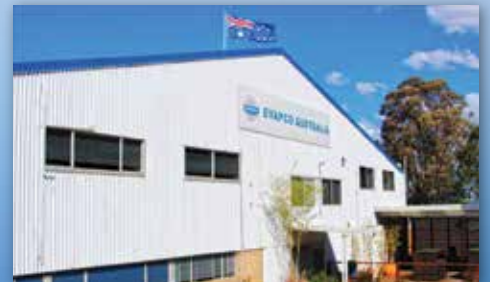
EVAPCO Australia (Pty.) Ltd. Riverstone, NSW Australia
